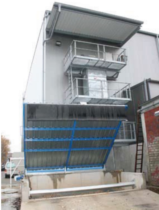
Fig. 4 The truck discharge bunker with ground level access feeding the double belt conveyor by means of a discharge conveyor.
